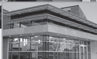
Renovated Residence Halls
